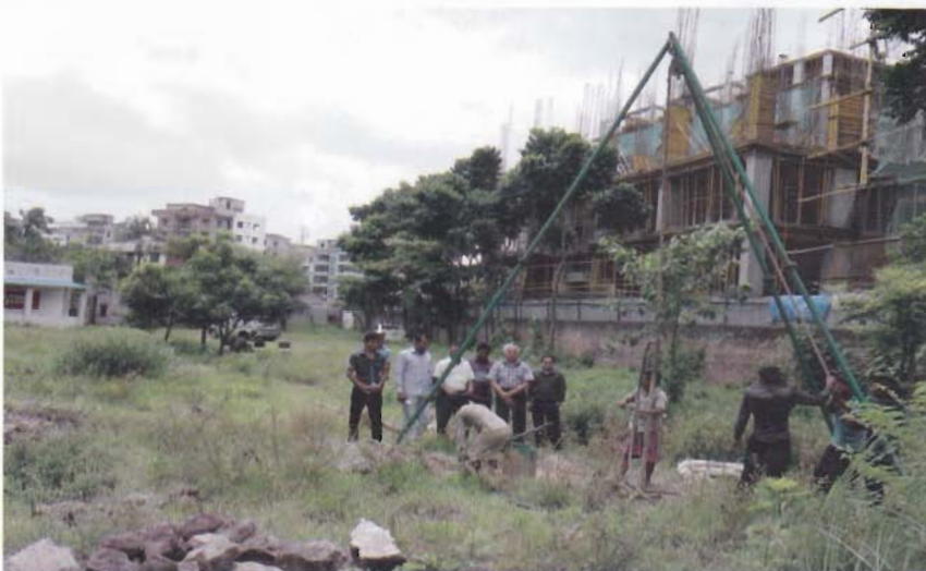
Vice Chancellor Dr. Profulla C. Sarker along with others watching the beginning of construction work at the permanent campus of the University
